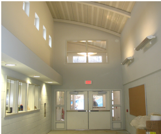
A view of the new interior lobby.
