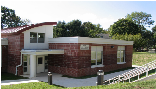
A view of the completed exterior.
