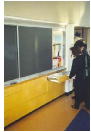
Storage behind and beneath chalkboard
